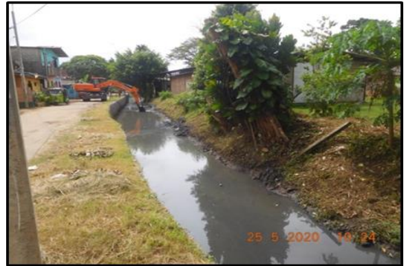
Maintenance work at Aramaya road canal
