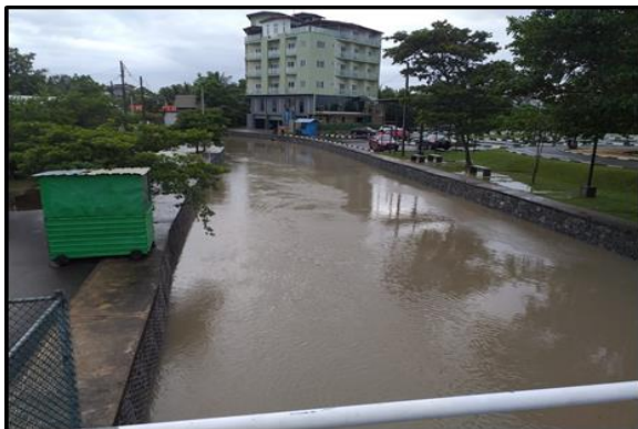
Bellanwila Canal Maintenance Work
