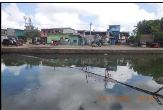
After cleaning the canal
