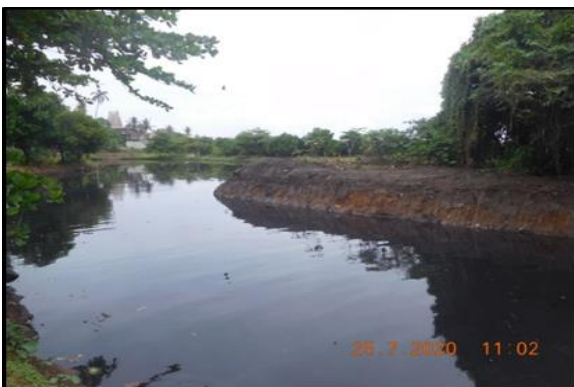
Maintenance work at Crow Island
