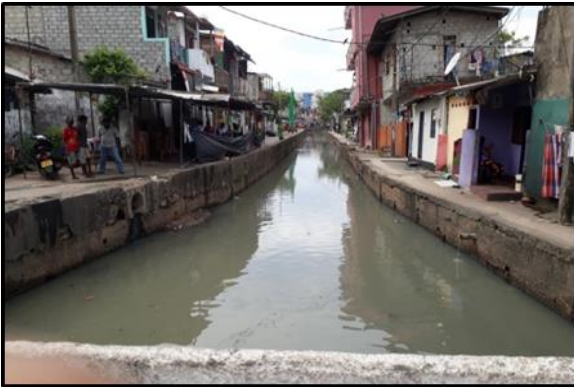
After cleaning the canal
