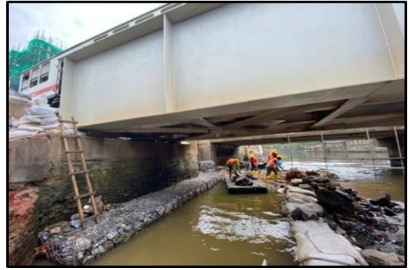
Canal Bank Improvement near Wallawaththa Outfall
