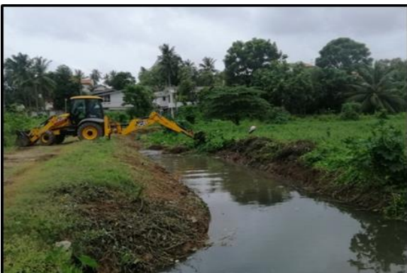
Surface Clearing Works of Akuregoda Peripheral Canal
