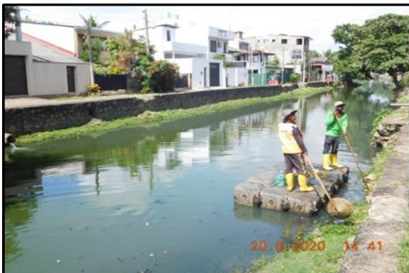
Cleaning the canal on progress
