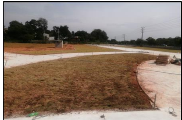
Construction work at Sandun Uyana Phase II
