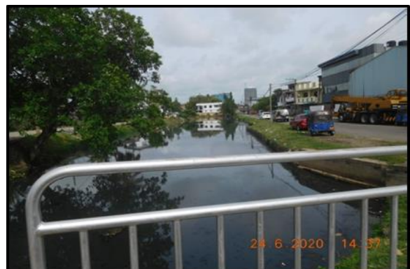
After cleaning the canal
