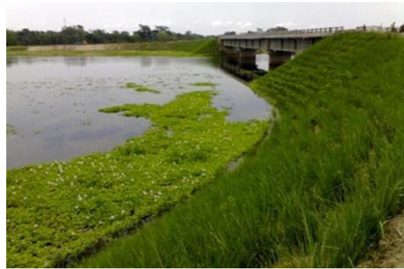
Canal bank restored with soft engineering techniques
