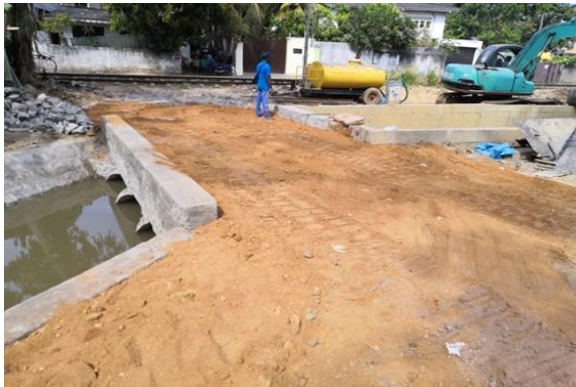
Hume Pipe Culvert and Rubble Pitching
