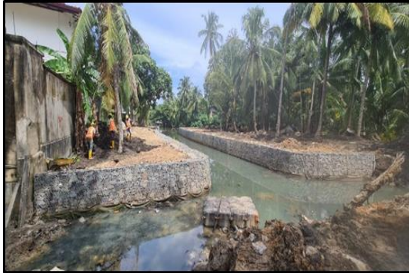
Construction work at Moragoda Ela
