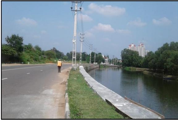
Gabion work at Lake Drive
