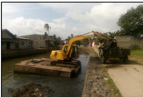
Dredging work near Isso wadiya area
