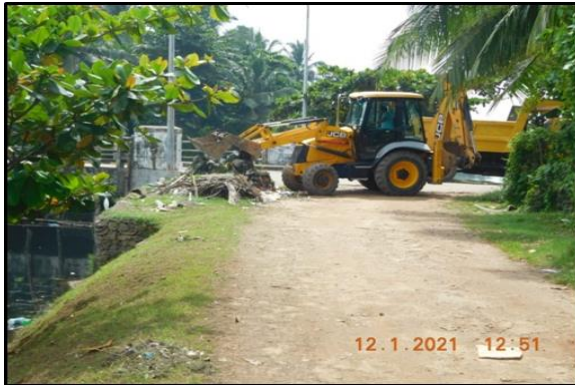
Garbage loading near N1 Canal
