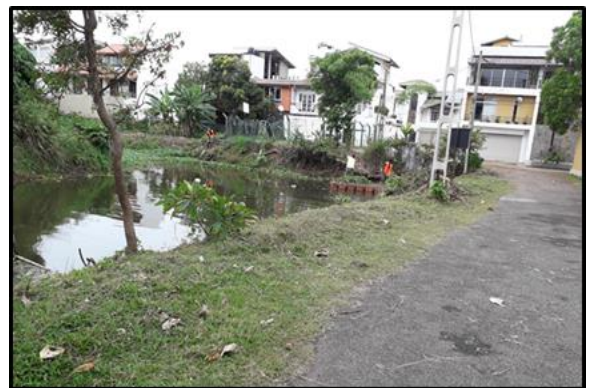
After cleaning the canal
