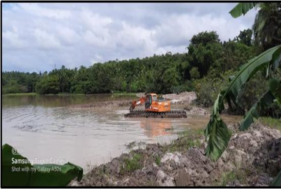
Desilting of Rannaka Wewa at Kotugoda (Stage I)
