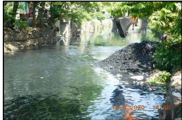
During cleaning of the canal
