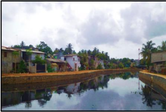
Kiththampahuwa Canal before and after the surface cleaning work
