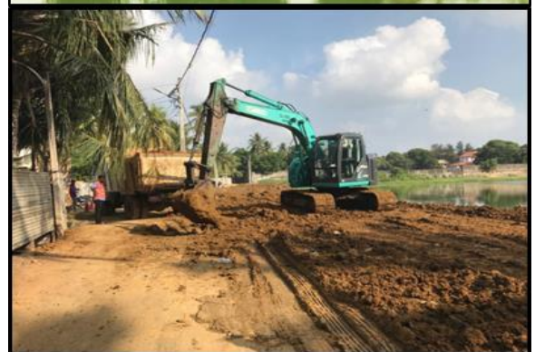
Construction work at Jaffna
