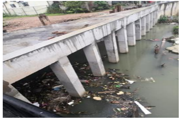
Outlet Structure at Rubber watta Wewa
