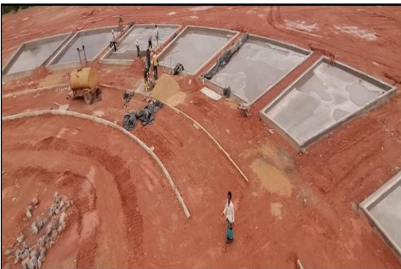
Construction work at Sandun Uyana Phase I
