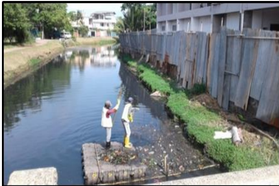
During cleaning of the canal
