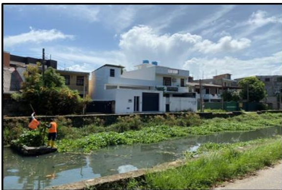
During cleaning of the canal
