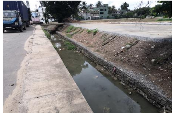
Gabion Work at the Earthen Canal Bed
