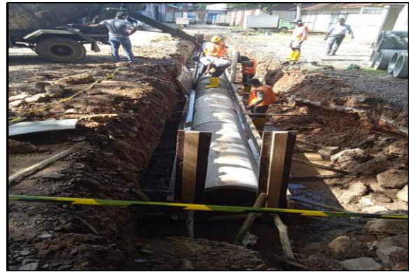
Storm water disposal system-Sangaraja Mw
