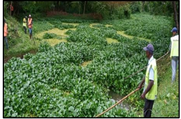
During cleaning of the canal
