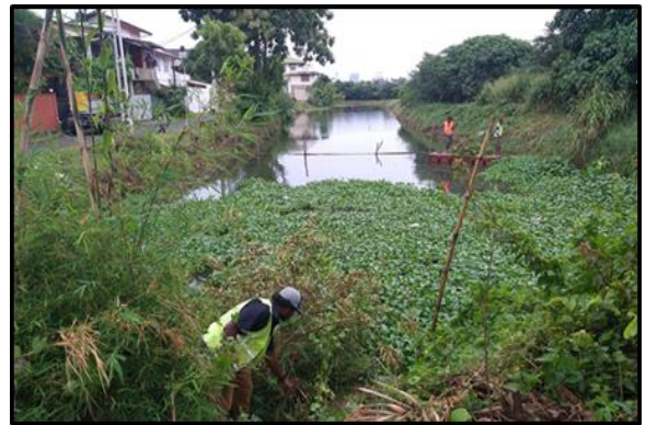
During cleaning of the canal
