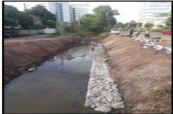
Drainage Improvement Work Robert Gunawardane Mawatha
