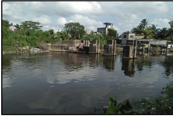
Kalu oya near Hekitta Log gate- Before and after cleaning
