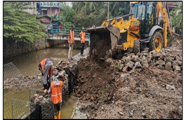
Gabion rectification works -Badowita Canal
