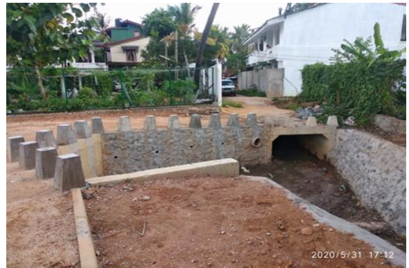
Finishing works to allow Public use of Manel Mawatha Wewa
