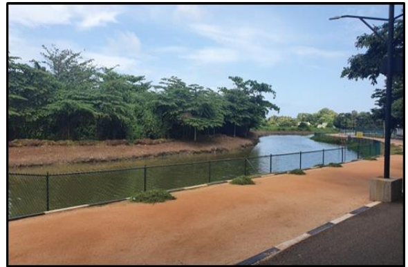
Bellanwila Walk path Maintenance Work
