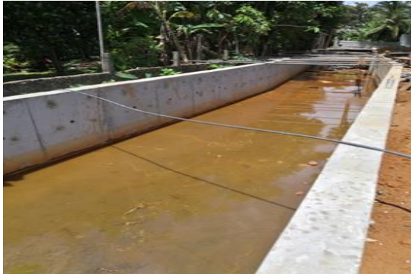
Ranasinghe Mawatha Canal Improvement Works
