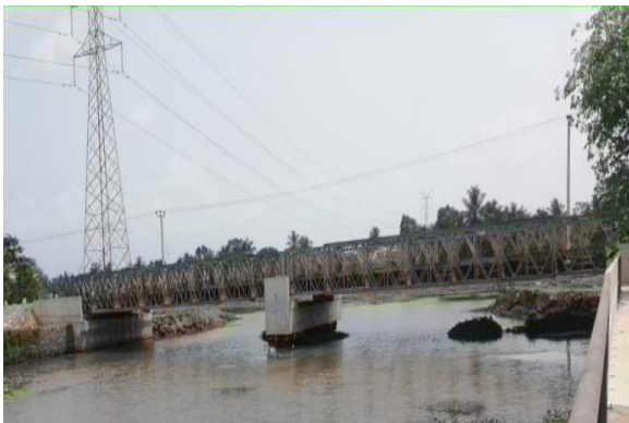
Maha Ela Bridge (40m Span)
